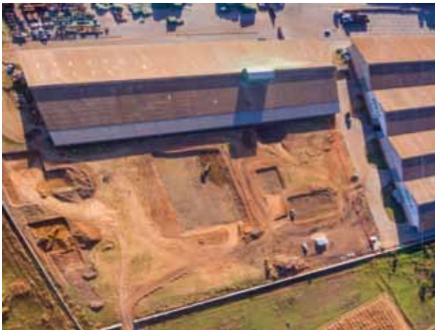
Aerial view of Seed Drying Plant construction
