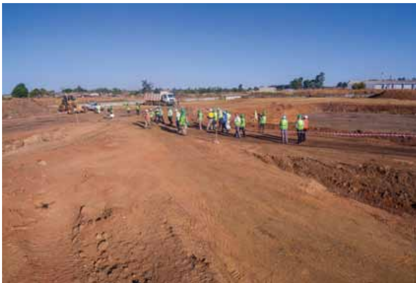
Inspection of construction site by Seed Co Limited Senior Management
